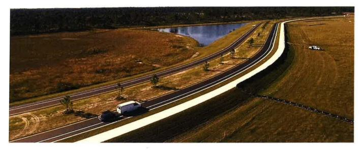
Stormwater design is integrated into the fabric of the infrastructure through innovative solutions that maximize construction efficiency and balance onsite earthwork. The stormwater management system is designed to mimic the natural systems and to recharge the groundwater table and minimize the erosive potential of runoff. Additionally, the stormwater system(s) will be designed considering adjacent development and the potential for shared uses as well as mixed uses (re-use / irrigation).
